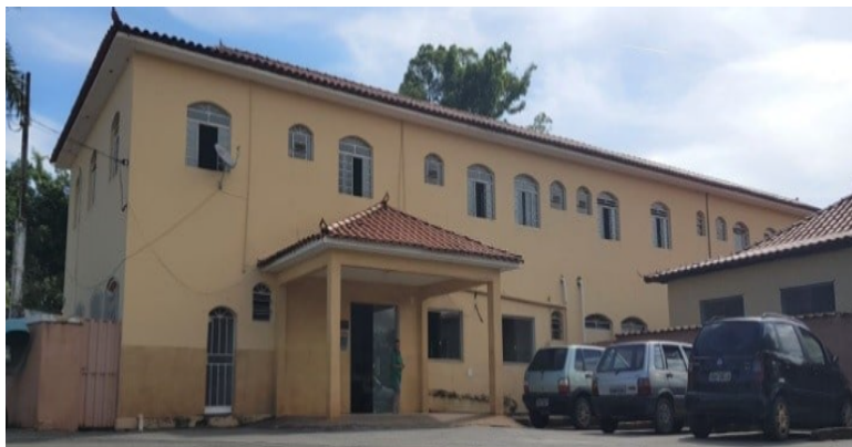
Hospital Municipal de Belo Vale/MG
