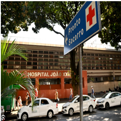
Hospital João XXIII
